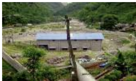
Figure IX. Small hydro powerhouse
