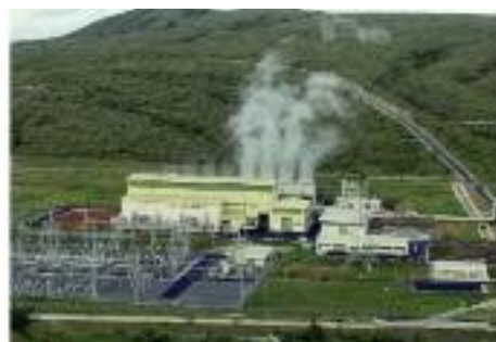
Figure II. Panoramic view of Olkaria II power plant in Kenya
