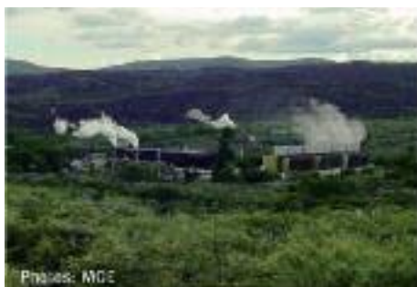
Figure I. The Olkaria I power station in Kenya
