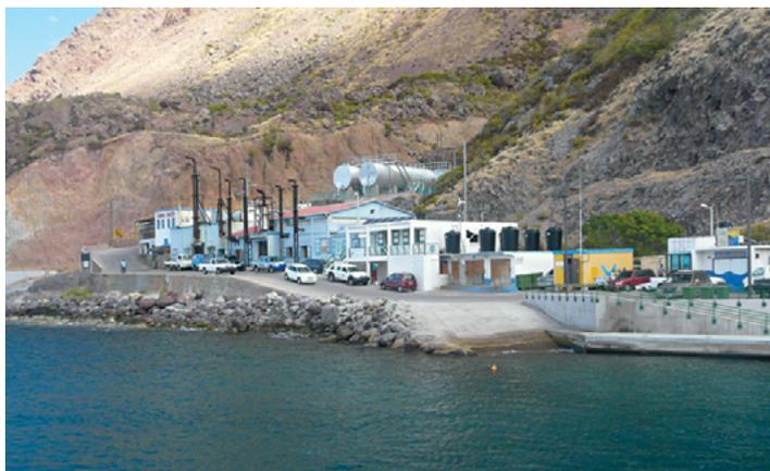
Saba's entire electric supply depends on a 4 MW diesel generator built near sea level.
