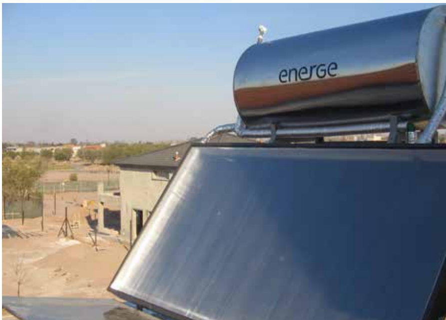
Roof-mounted solar water heater. (Credit: Wikipedia, Cachogaray)
