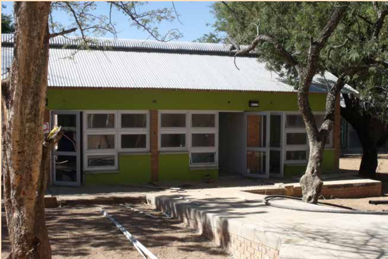
The design of a new South African health facility aims to curb cross-infection of patients with drug resistant TB using natural ventilation. (Credit: Council for Scientific and Industrial Research in South Africa)
