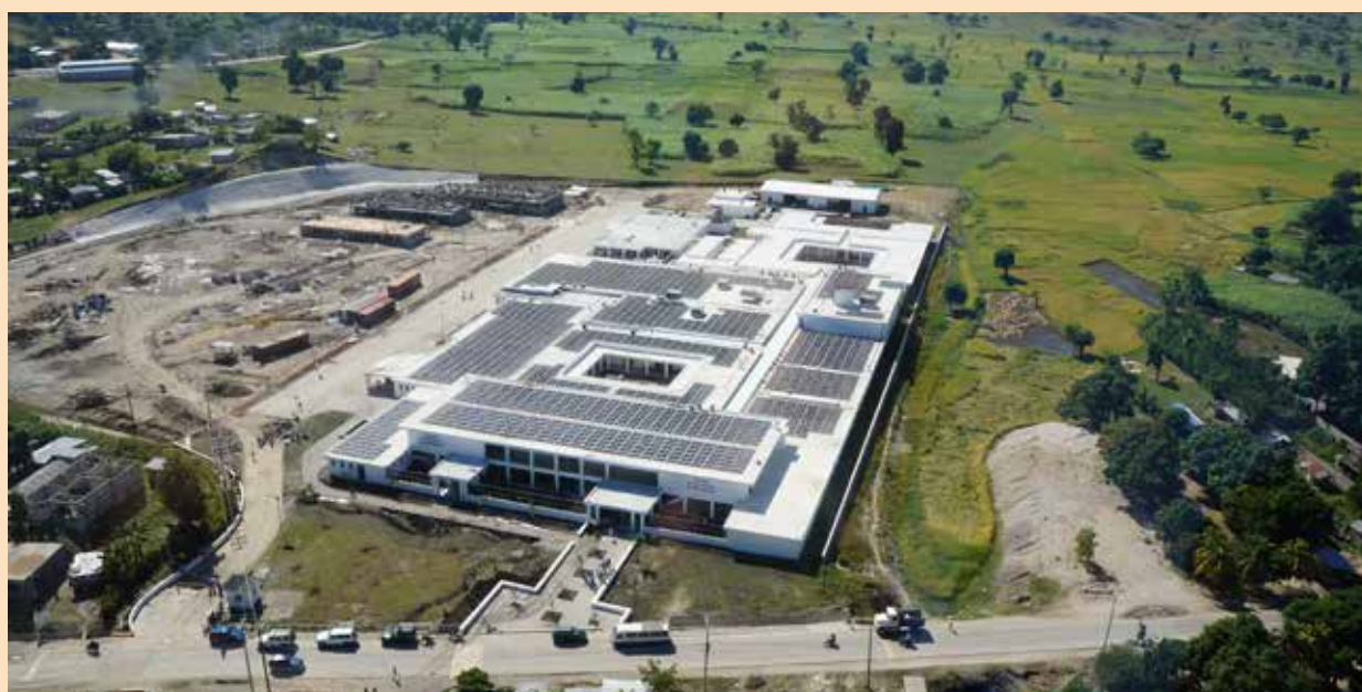
An aerial view of University Hospital of Mirebalais, Haiti reveals 1,800 solar panels on the hospital's rooftop. (Credit: Rebecca E. Rollins/Partners in Health)
