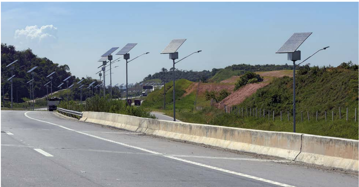
Solar panels used for street lighting in the Metropolitan Ring of Rio de Janeiro
